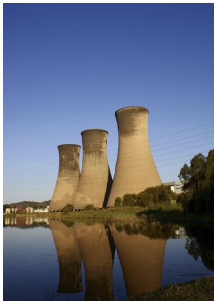
Example of cooling towers
